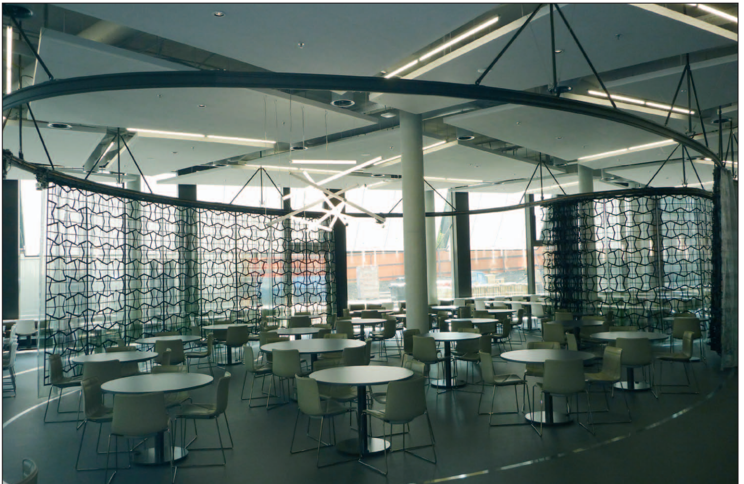
//Photo: Gerriets / FHNW Brugg – Switzerland / STUDIO E tracks with 5 FRICTION-DRIVE motors
